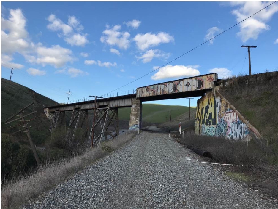
Photograph 1. View of southwest side of Altamont Pass UP Bridge (33C0013) from SPRR ROW, camera facing north, February 6, 2019.
