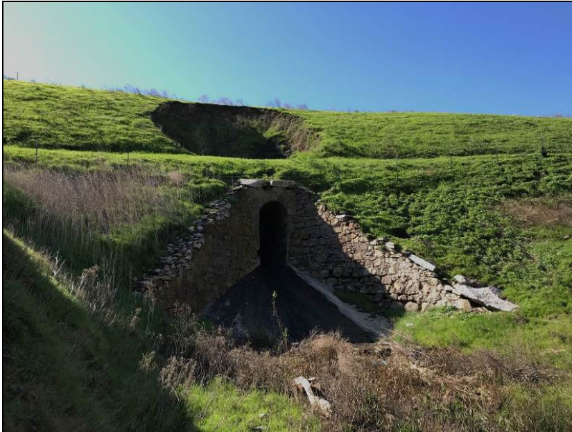
Photograph 9. Culvert 6 (northeast side), camera facing southwest, February 6, 2018.
