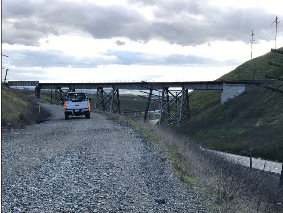
Photograph 2. View of northeast side of 33C0013 from SPRR ROW, camera facing southwest, February 6, 2019.
