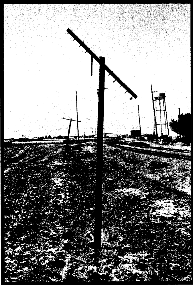
Pole 13, view west. Roll RR4, Fr.6. 9-04-02, 1:23 PM.
