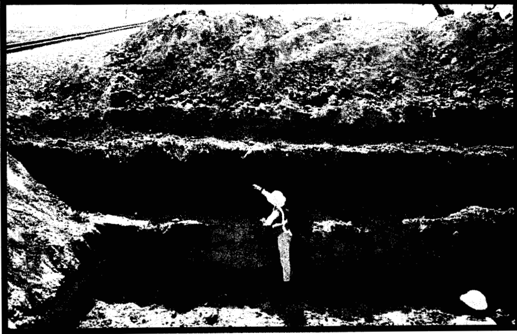
Utility bore pad; profile with ditch. Roll RR2, Fr.6. 8-13-02, 4:20 PM.
