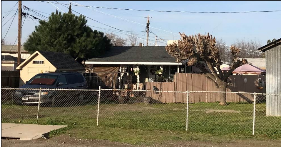
Photograph 4. East elevation of 52 East 4th Street, camera facing west, February 7, 2019.
