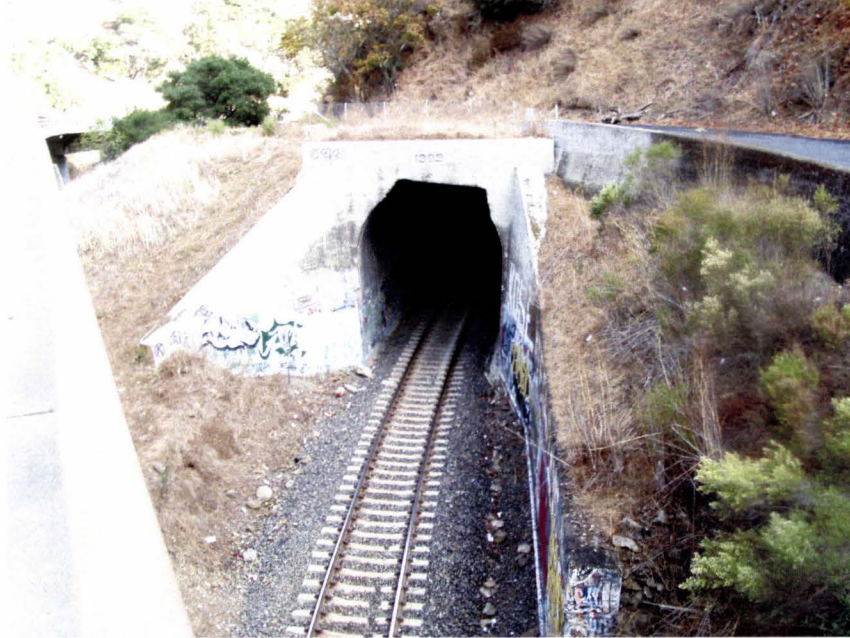
Western Pacific Railroad Tunnel #2, view facing east from east edge of Bridge 33-0039 on State Route 84.
