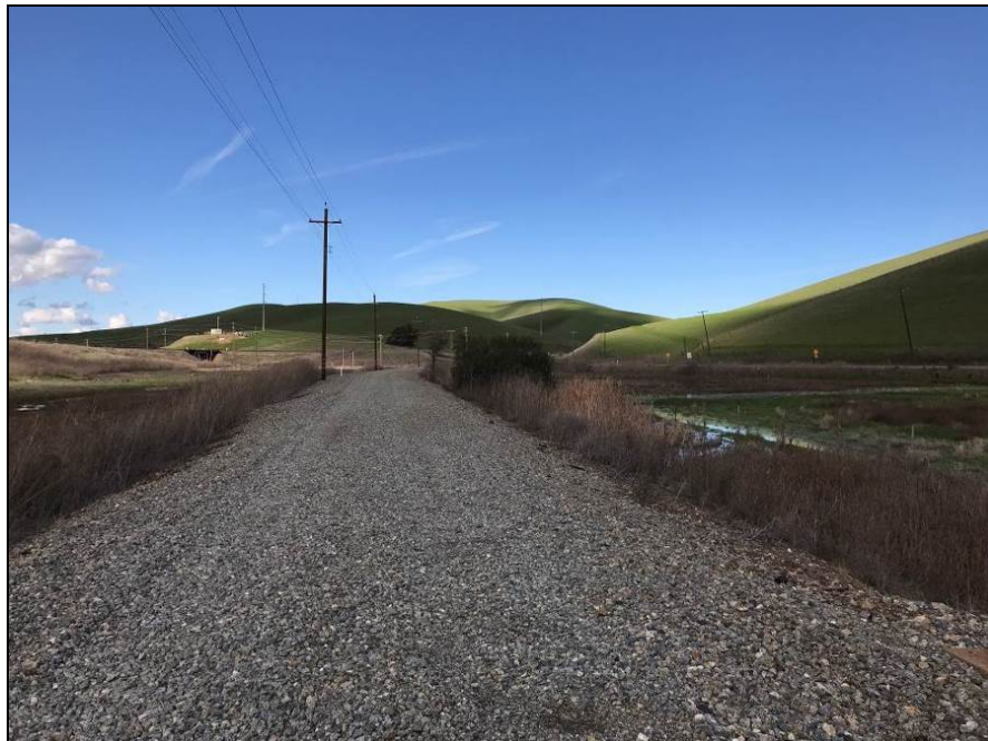
Photograph 25. Railroad Segment 5, camera facing northeast, February 6, 2018.
