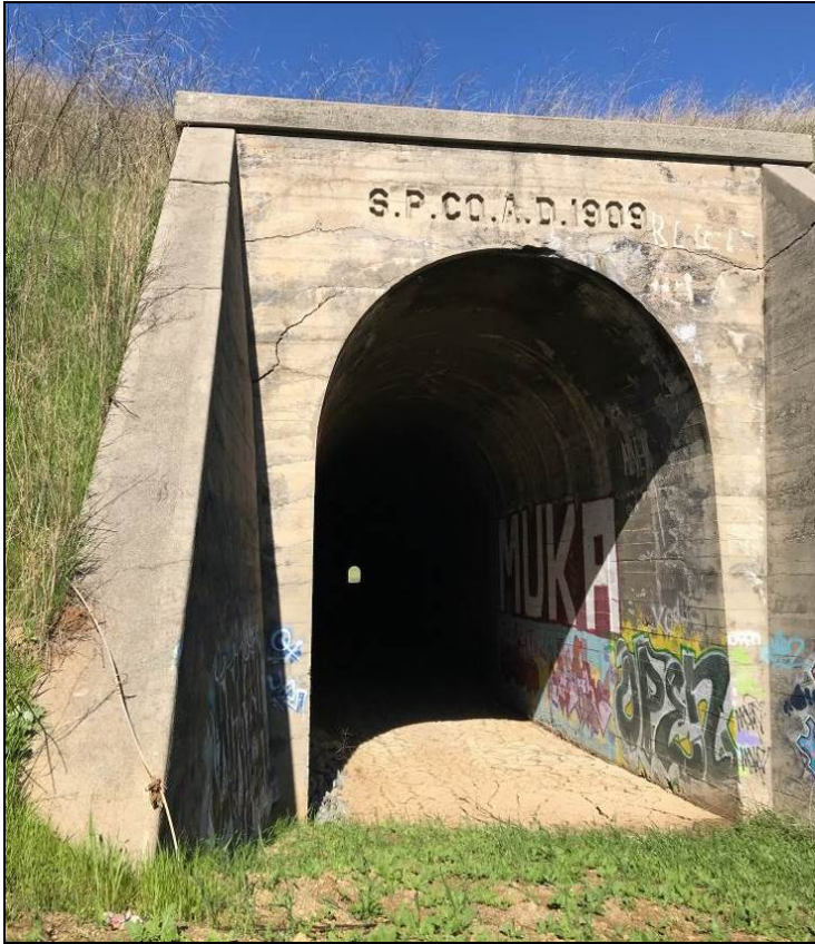
Photograph 33. Detail view of south side of tunnel, camera facing north, February 6, 2019.
