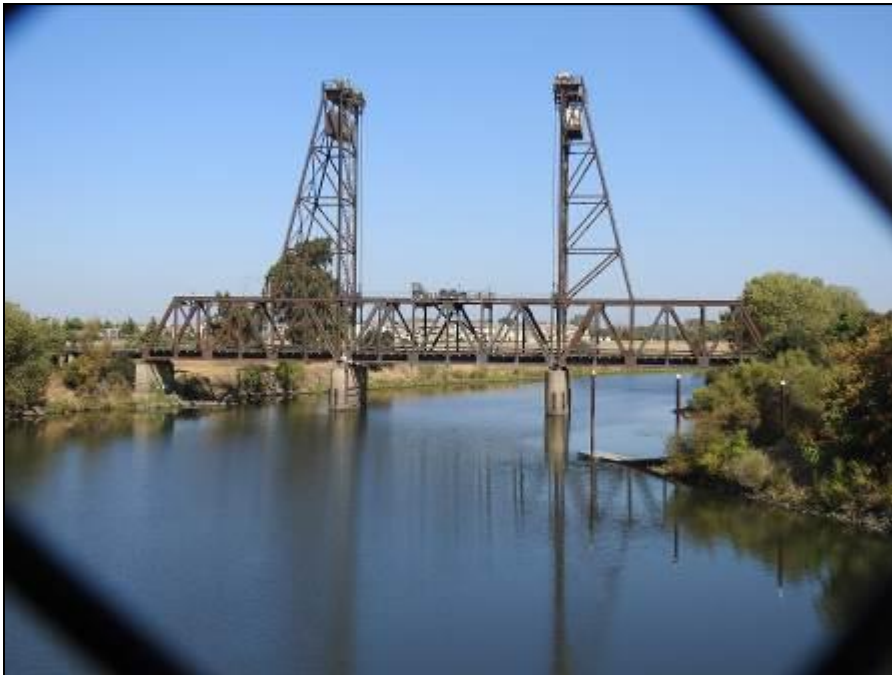
Photograph 1. Mossdale Railroad Bridge, camera facing north, September 20, 2016.
