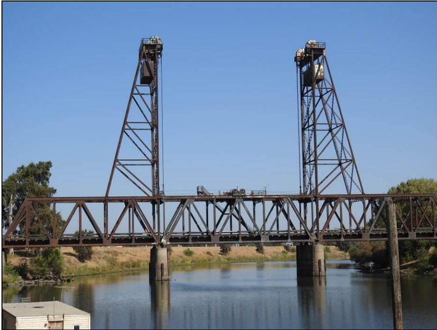
Photograph 2. Mossdale Railroad Bridge, camera facing north, September 20, 2016.
