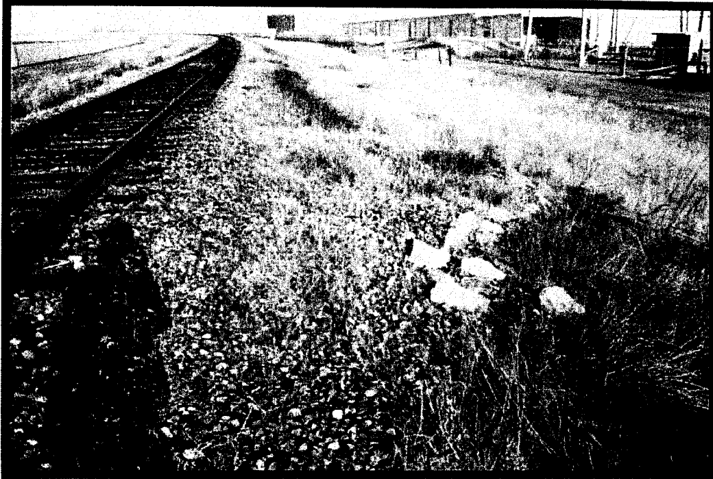
Western switch station. Retaining wall to platform on north side of tracks. View west. Roll RR2, Fr.20. 8-19-02, 7:50 AM.
