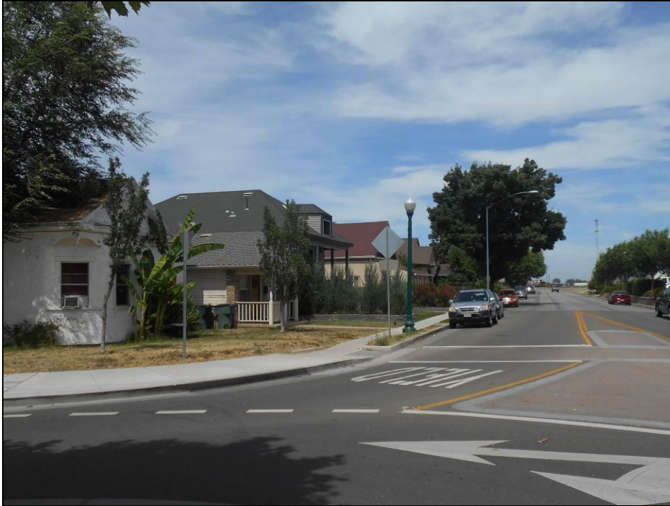
Photograph 3. Contributing Residences within Tracy Historic District near the Intersection of 6th Street and D Street, camera facing northeast, June 8, 2016 (PHOTO #1329)
