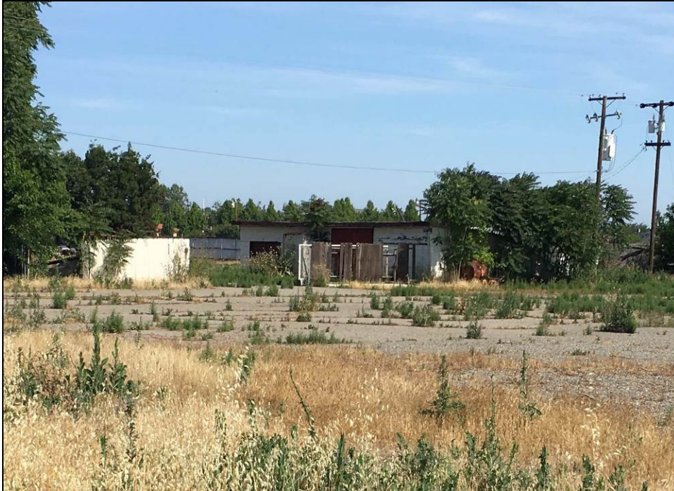
Photograph 3. South and east sides of office and storage building, camera facing northwest, February 7, 2019.
