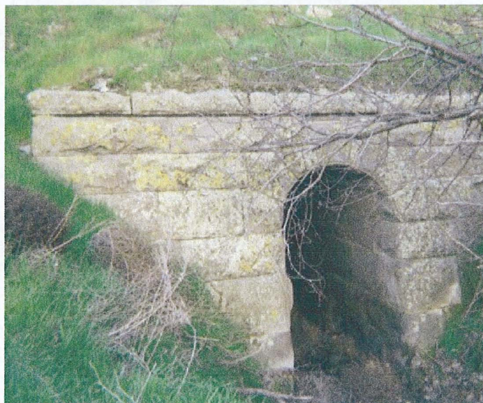
Central Pacific Railroad Culvert, view facing east,
