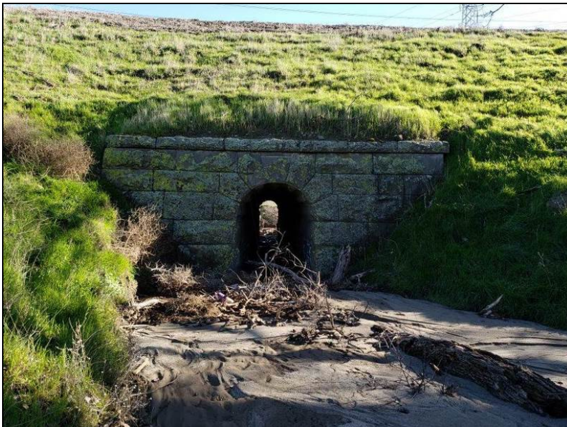
Photograph 2. Culvert 1, camera facing northeast, February 6, 2018.
