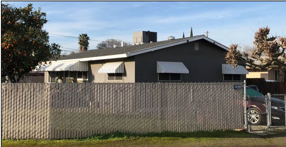
Photograph 2. Façade and north elevation of 50 East 4th Street, camera facing southwest, February 7, 2019.
