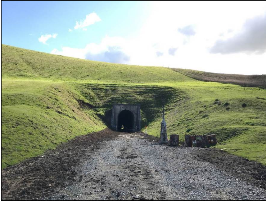
Photograph 35. North side of tunnel with Signal 4 and barrels at center, camera facing south, February 6, 2019.
