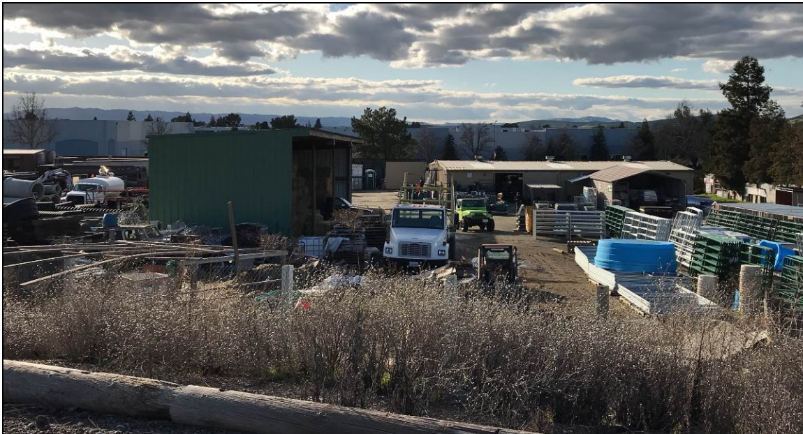
Photograph 2. East side of store/office building on right with Storage Shelter 1 abutting the east side, at right. North and east sides of Storage Shelter 3, at left, portion of mobile office at far left, camera facing west, February 6, 2019.
