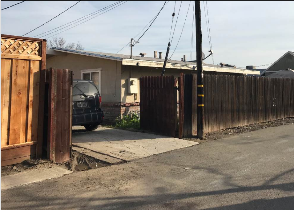
Photograph 2. West and south sides of 26 East 4th Street, off of King Alley, camera facing northeast, February 7, 2019.
