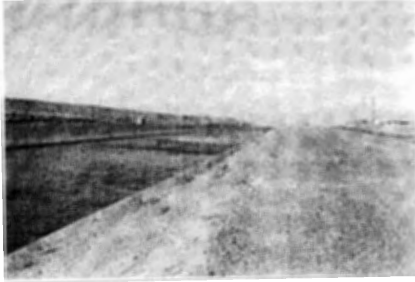
Two views of the Delta-Mendota Canal looking north.
