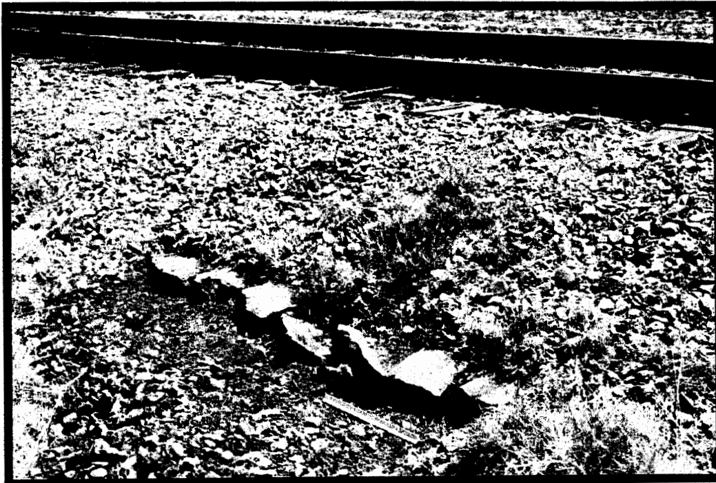
Stone retaining wall, north side of tracks at cross-section; 1ft. scale foreground; view SE. Roll RR2, Fr.2. 8-06-02, 1:45 PM.
