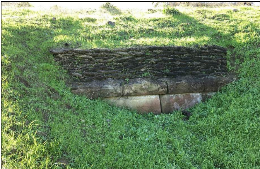
Photograph 8. Culvert 5 (north side), camera facing south, February 6, 2018.
