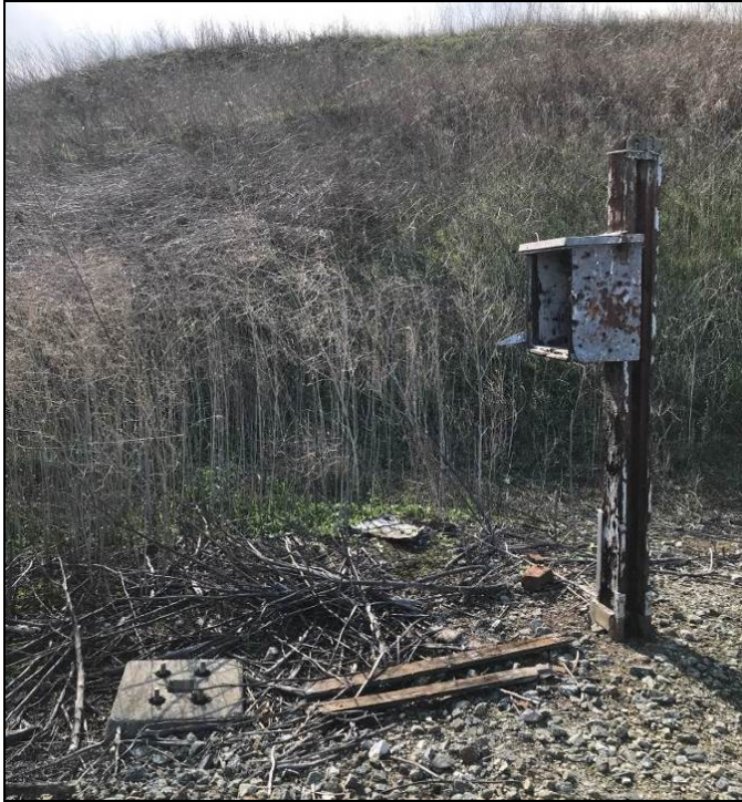
Photograph 31. Signal 5, utility box, and footing east of Altamont, camera facing southwest, February 6, 2019.
