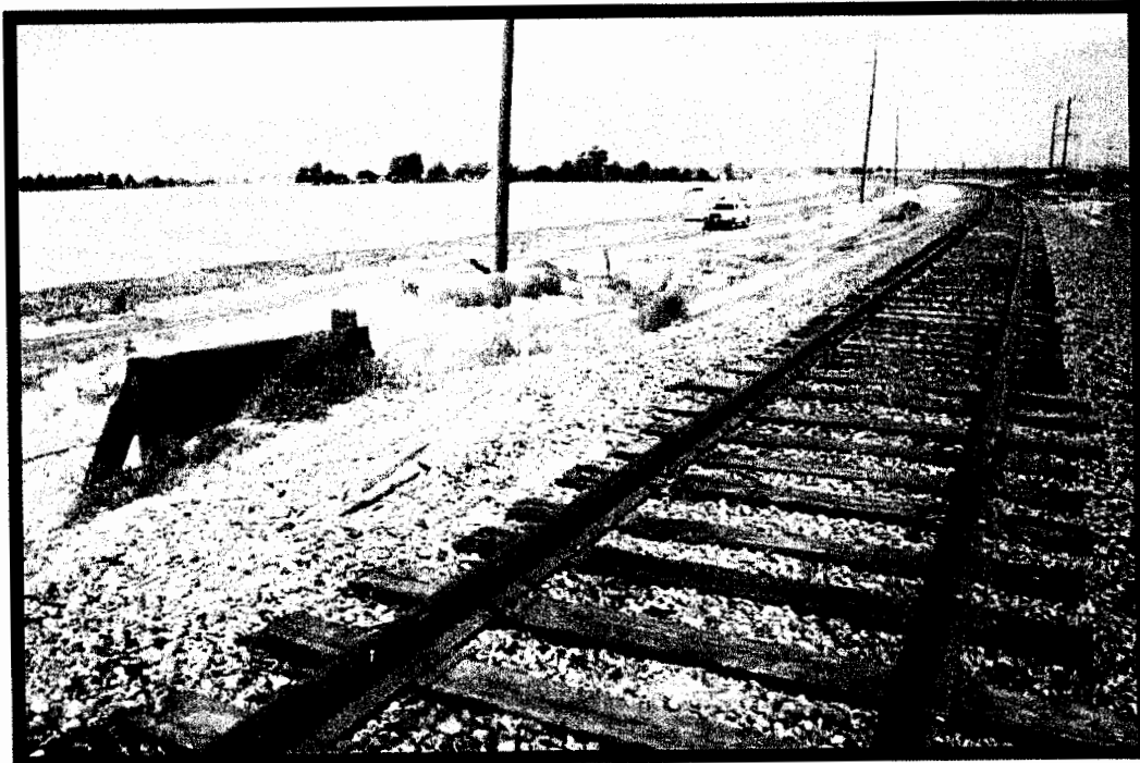
Section car turnout, View NE. Roll RR2, Fr.26. 8-19-02, 2:05 PM.
