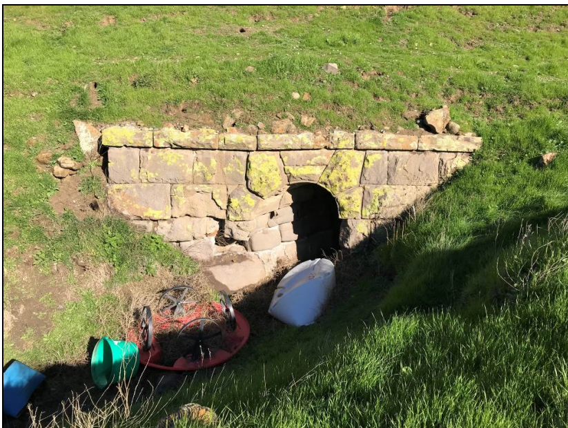
Photograph 6. Culvert 4 (south side) with keystone, camera facing north, February 6, 2018.
