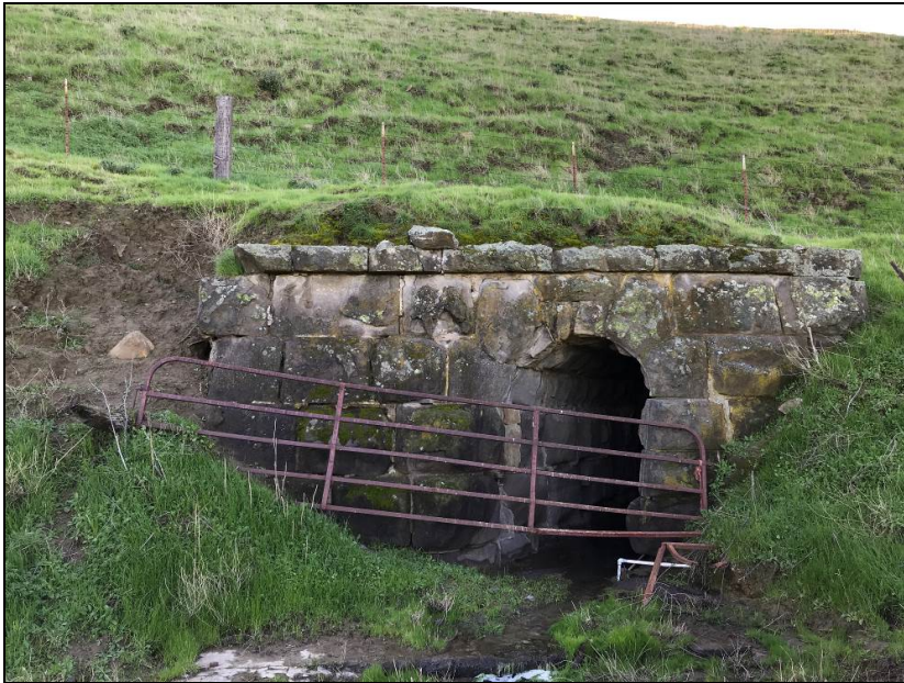
Photograph 5. Culvert 4 (north side), camera facing south, February 6, 2018.
