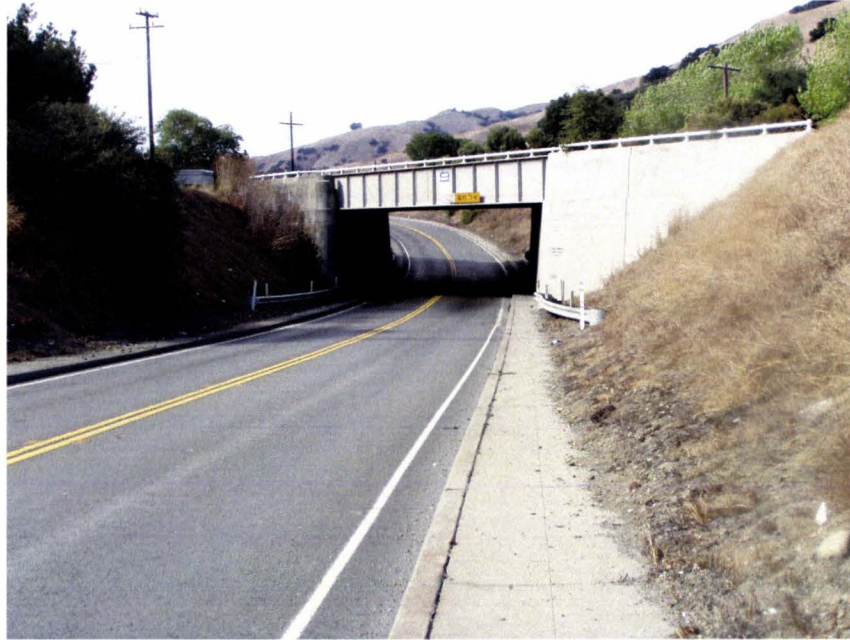
East side of Bridge 33-0042, camera facing west along SR 84.
