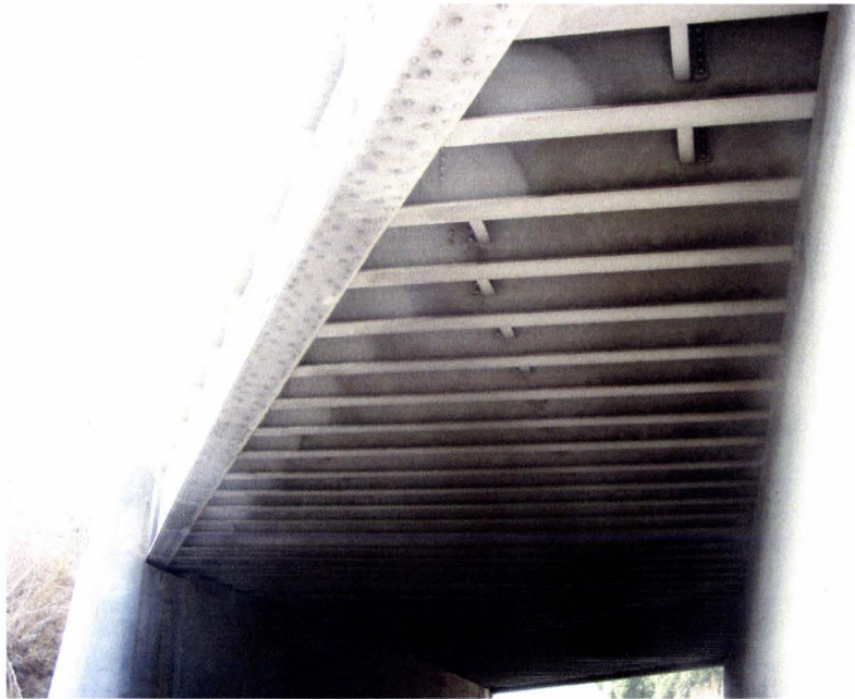
Detailed view of deck underside.
