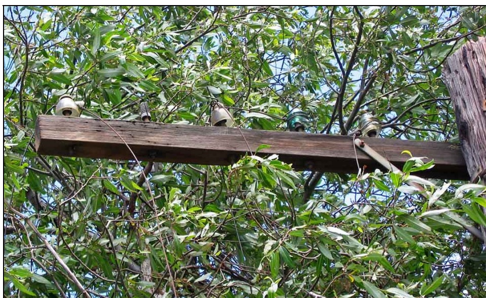
Close-up of right half of utility pole crossarm showing remaining insulators.
