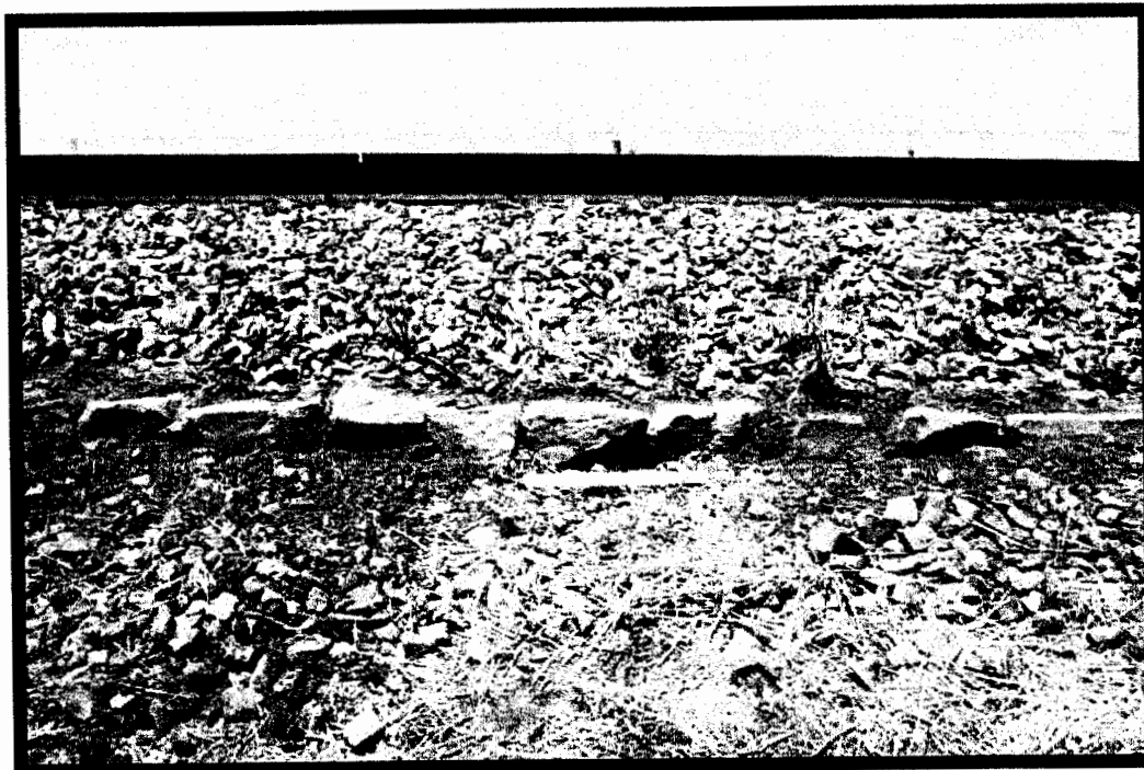
Stone retaining wall, south side of tracks at cross-section; 1ft. scale foreground; view north. Roll RR2, Fr.1. 8-06-02, 1:40 PM.
