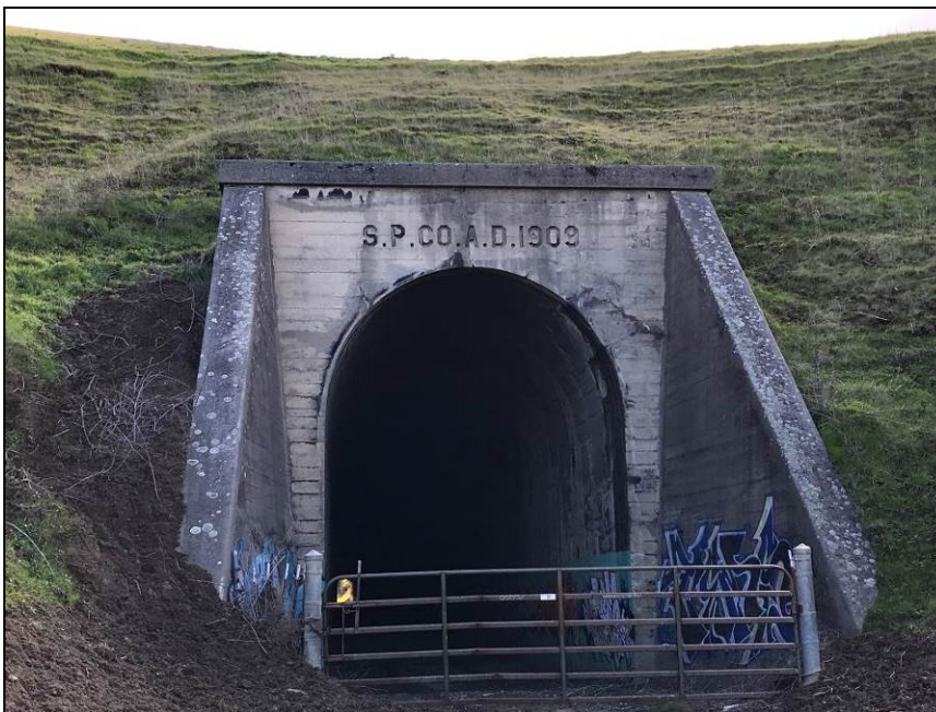
Photograph 36. Detail view of north side of tunnel, camera facing south, February 6, 2019.
