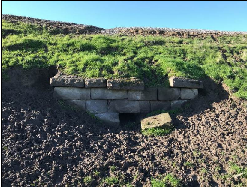
Photograph 3. Culvert 2, camera facing southwest, February 6, 2018.
