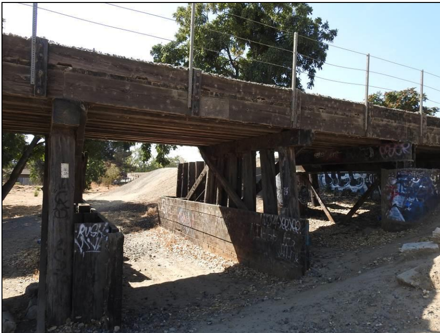
Photograph 3. East foundation, camera facing north, September 20, 2016.
