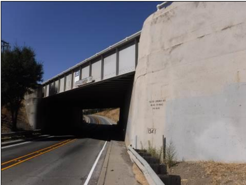
Photograph 5. Bridge 33-0042 / Silver Springs Underpass, camera facing west, September 22, 2016 (Photo #861)
