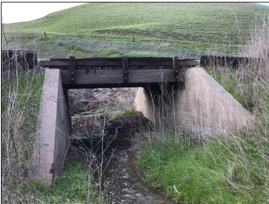
Photograph 18. Culvert 10 concrete culvert with wood deck, camera facing northwest, February 6, 2018.
