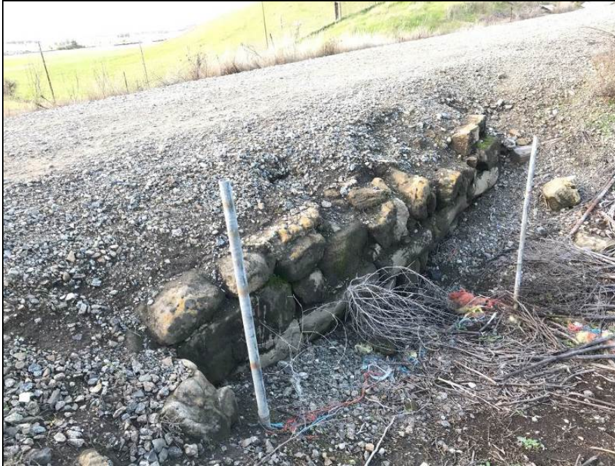
Photograph 21. Culvert 13 (east side), camera facing north, February 6, 2018.
