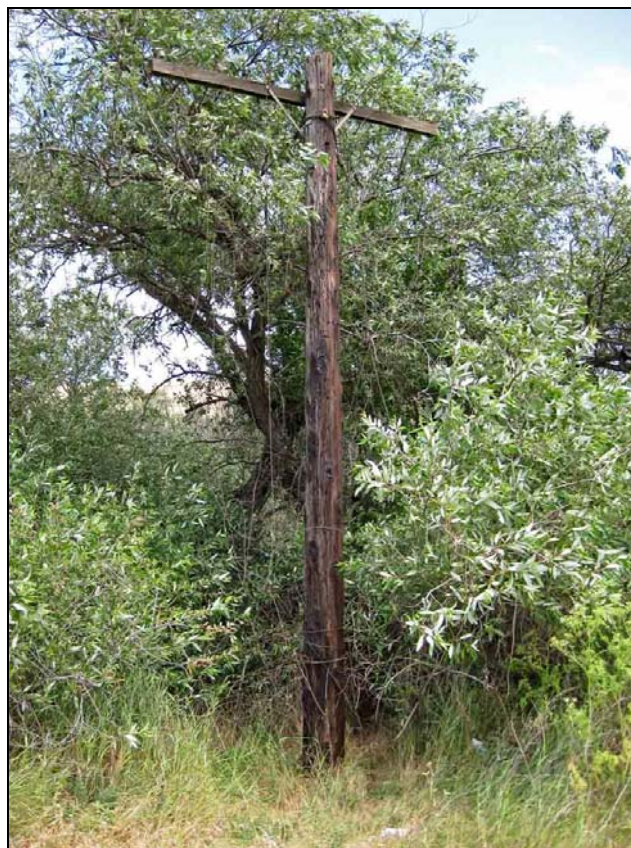
Utility pole near Altamont Creek, facing east.
