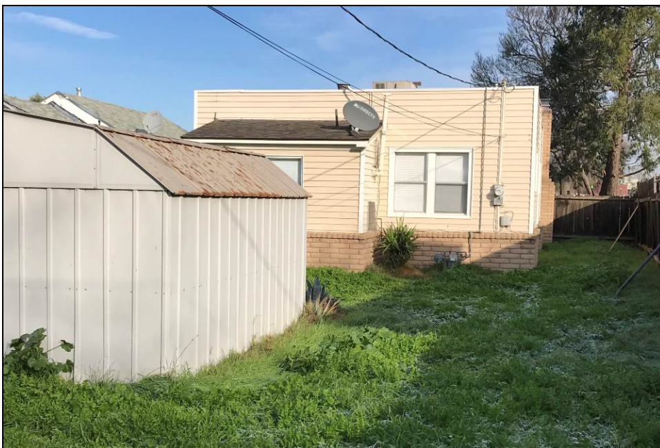
Photograph 3. South side of 16 West 4th Street, camera facing north, February 7, 2019.
