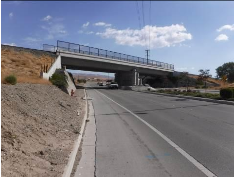
Photograph 6. Circa 2005 Greenville Road Bridge, camera facing south, September 22, 2016 (Photo #882)
