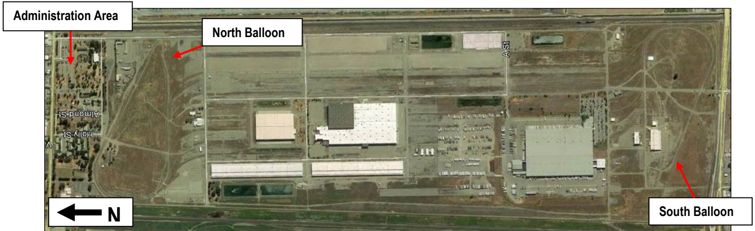
Photograph 4. Current Aerial Image of the Sharpe Army Depot and Condition of Original Railroad System (GoogleEarth May 2017; notations added by AECOM)
