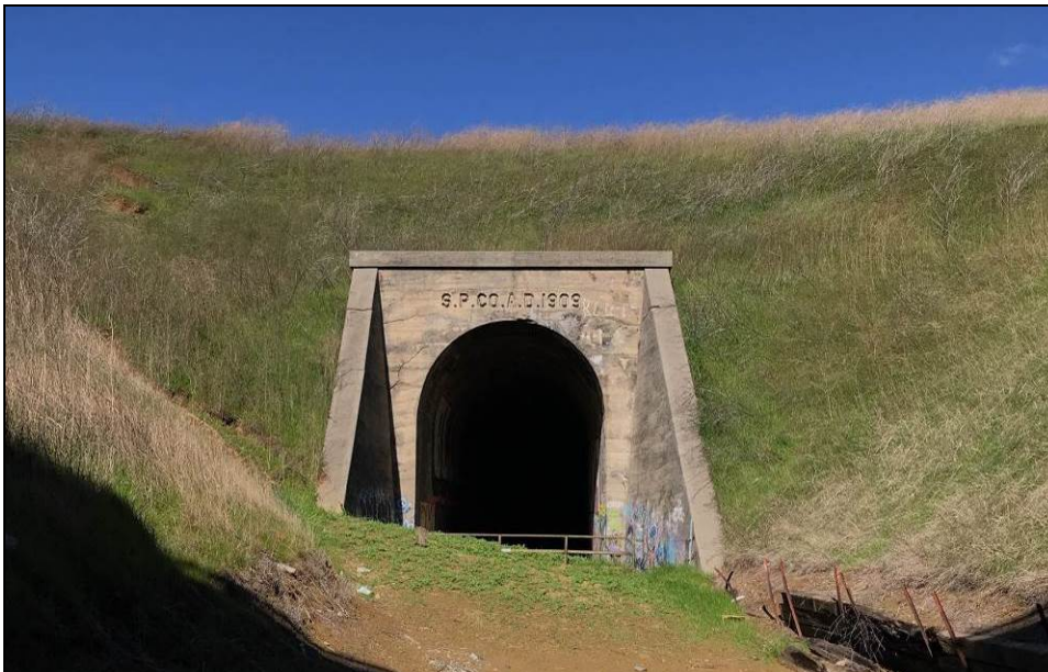
Photograph 32. South side of tunnel, camera facing north, February 6, 2019.
