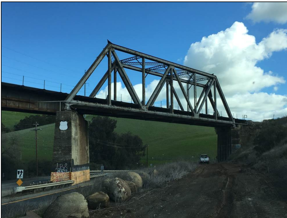
Photograph 3. View of southwest side of 33C0109 from SPRR ROW, camera facing southwest, February 6, 2019.
