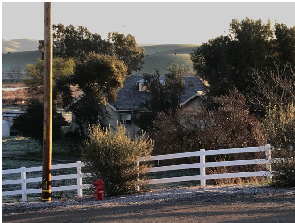
Photograph 2. West side of residence, camera facing northeast, February 6, 2019.
