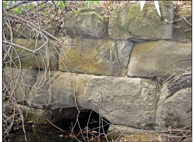
South end of culvert.
