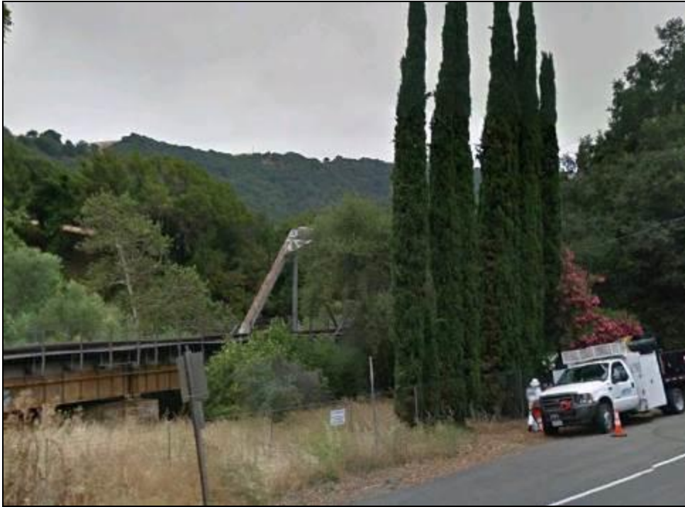
Photograph 2. Silver Springs Truss Bridge, camera facing southwest, Google Image Capture July 2015
