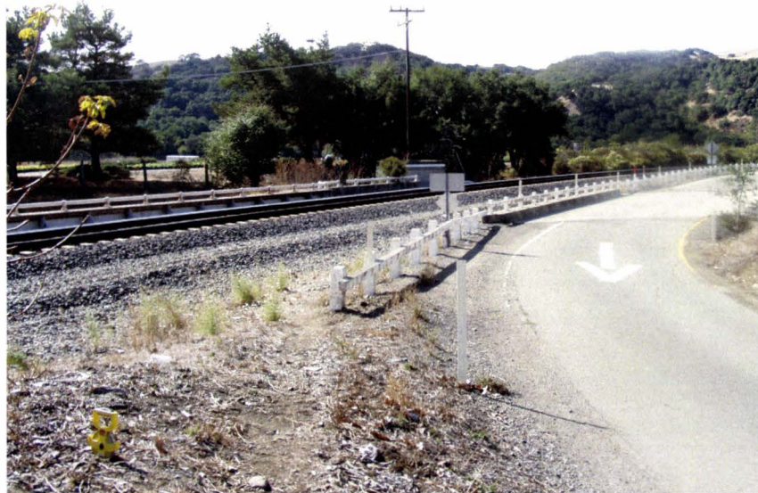
Deck view of Bridge 33-0042, camera facing southwest along SR 84 offramp (wich carries eastbound traffic into Sunol).
