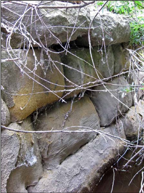
North end of culvert.
